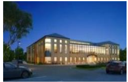
Rear View of Future Expanded Library
