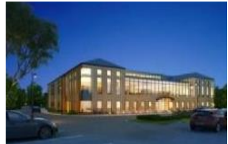
Rear View of Future Expanded Library
