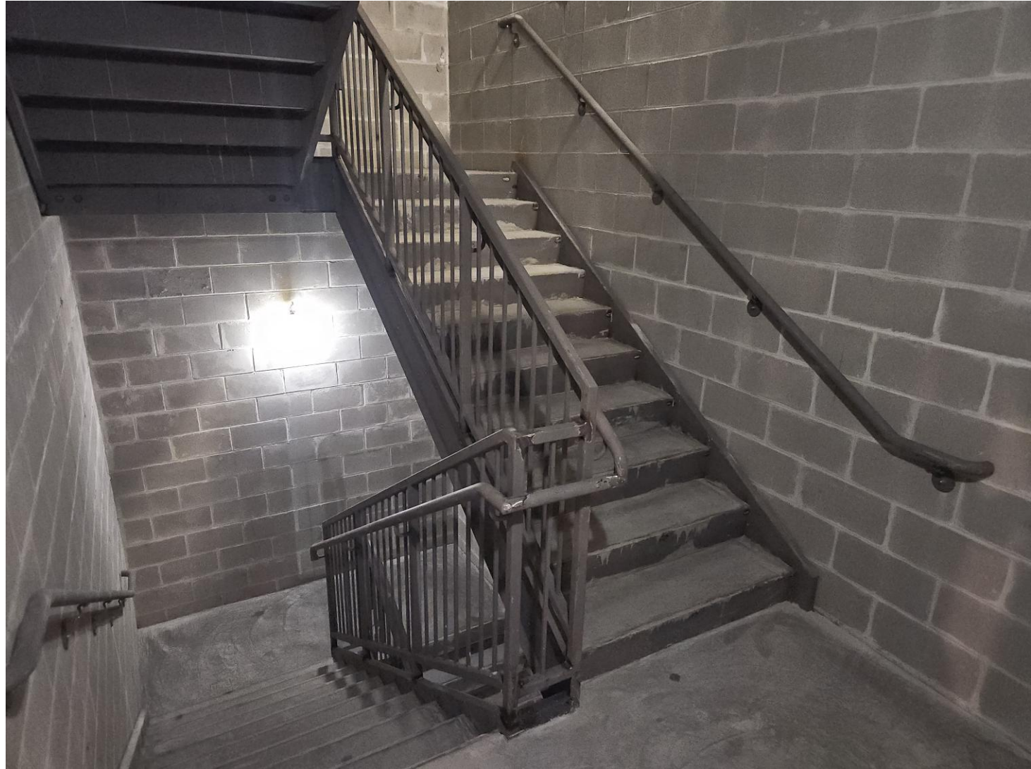
Interior Construction Progress, Stair C, August 2026
