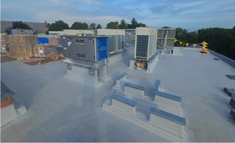
Roof Top Equipment Installation
