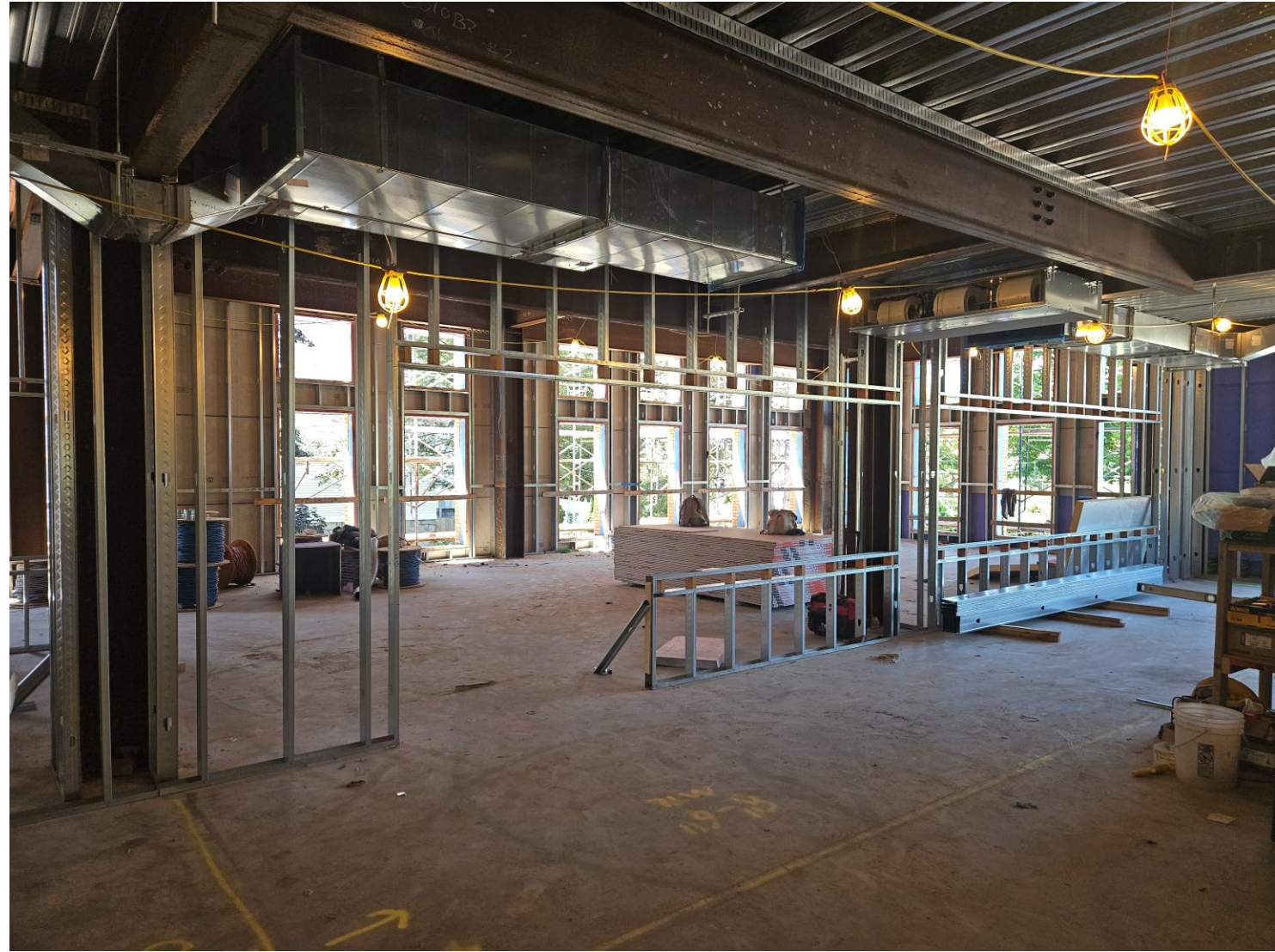
Construction Progress of Interior, August 2026
