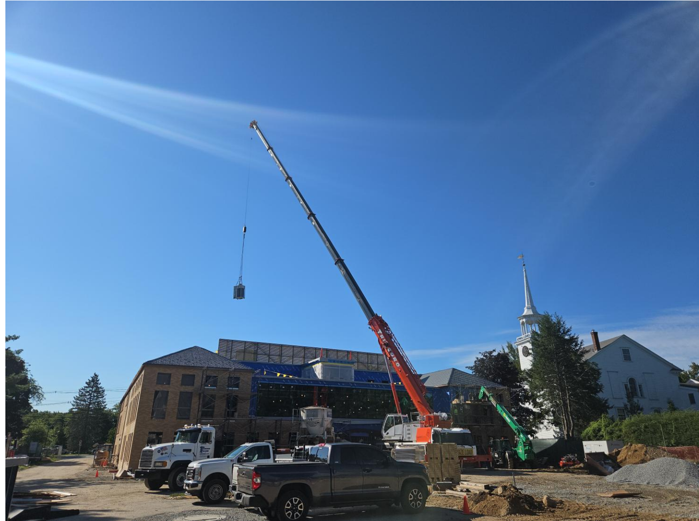
Crane delivering Rooftop Equipment, August 2026
