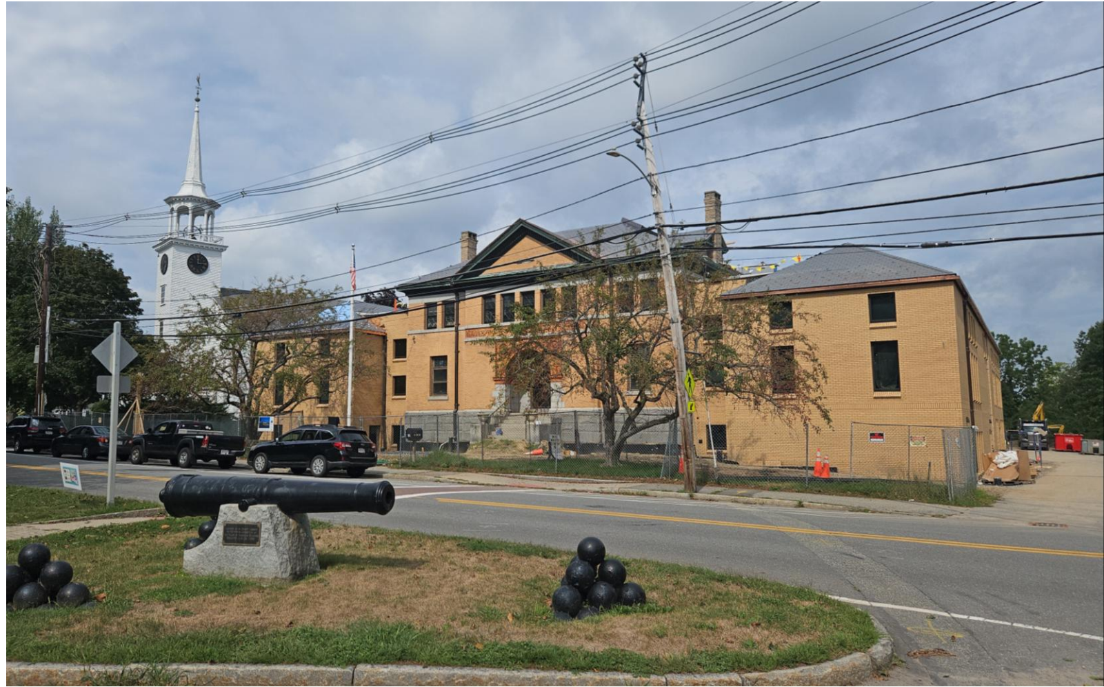
Construction Progress at Main Street Elevation, August 2026
