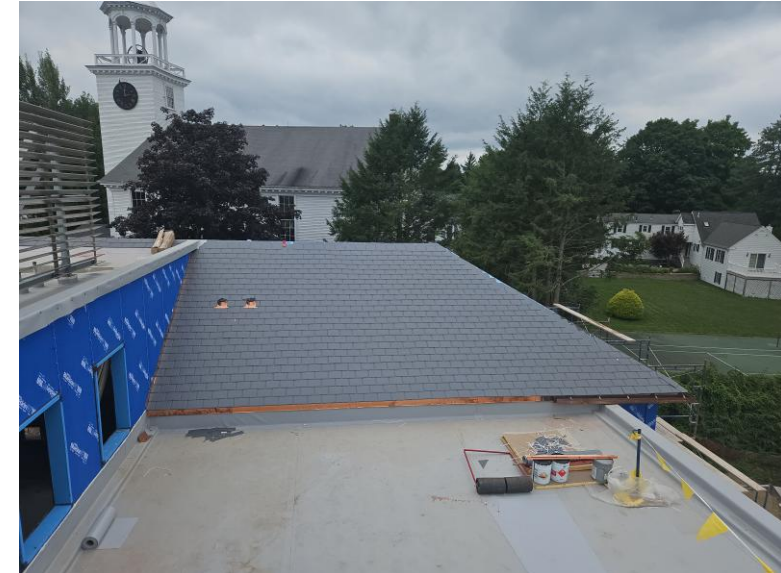
Roof Installation Progress
