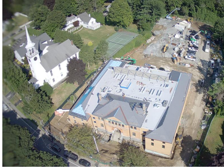
Roof Installation: Drone Footage, c/o Westford Police Dept
