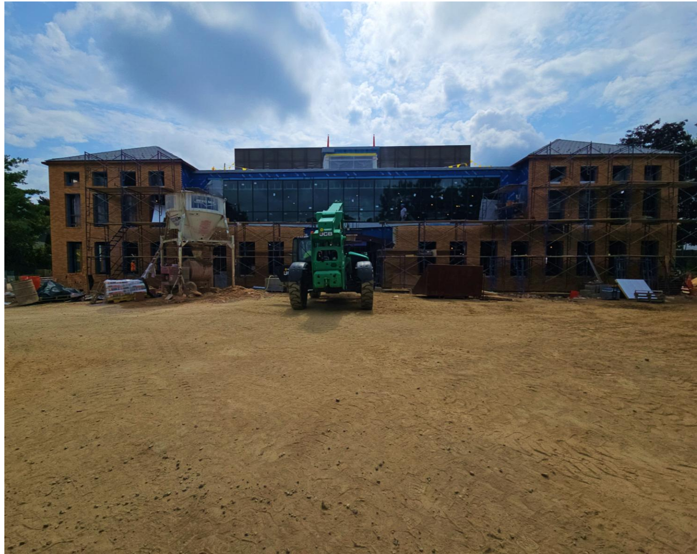
Construction Progress, Exterior Envelope, August 2026
