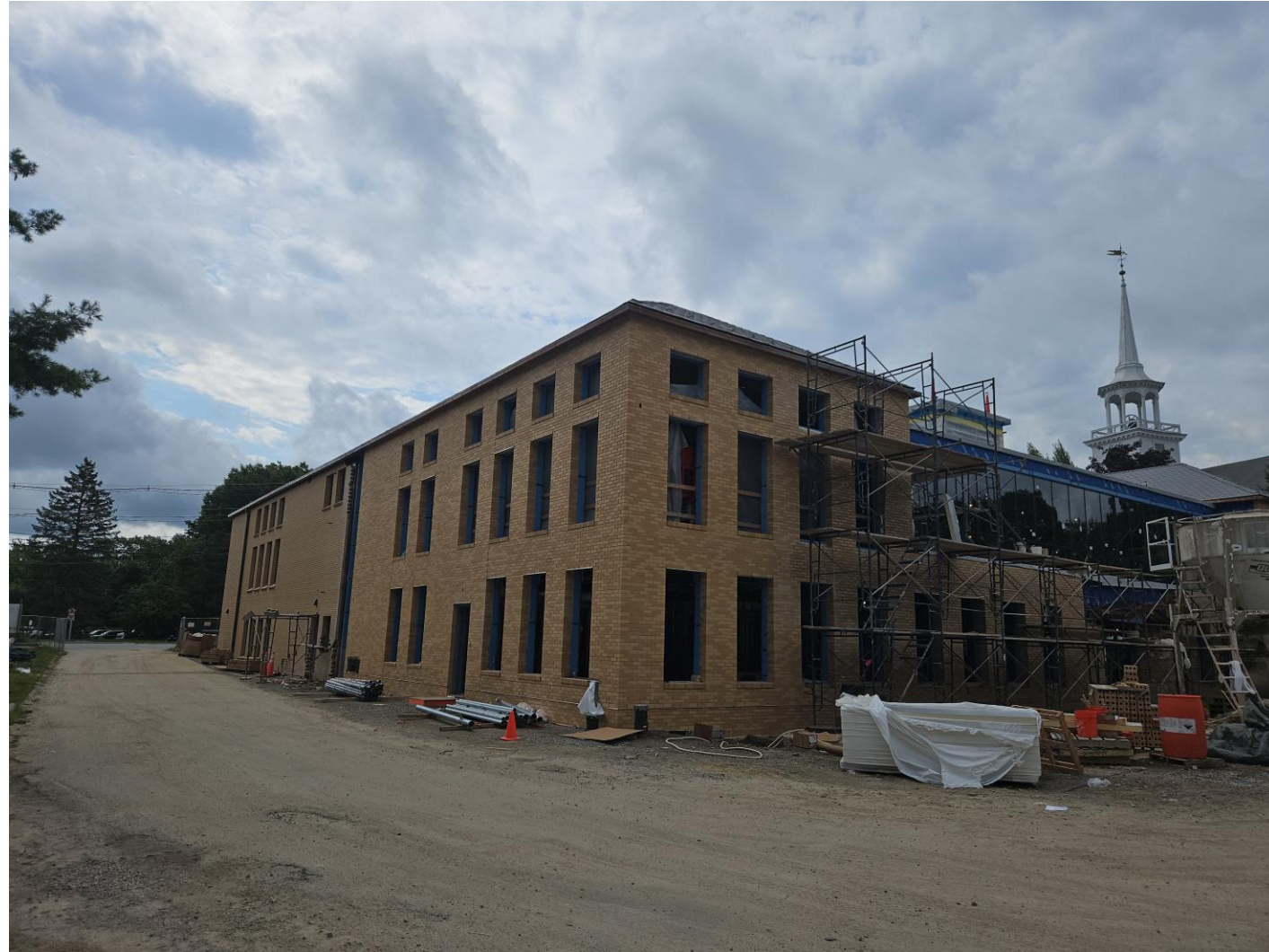
Construction Progress of New Facade, August 2026
